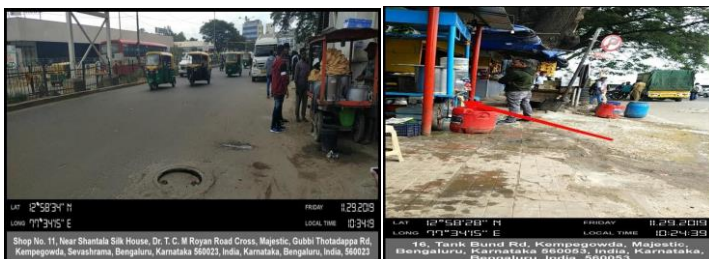
Fig 2A: Manhole at varying heights with respect to road surface
