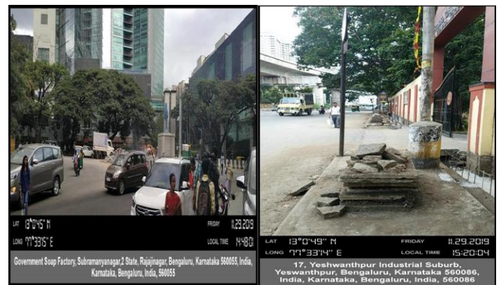
Fig 8: Road under construction, no road marking
