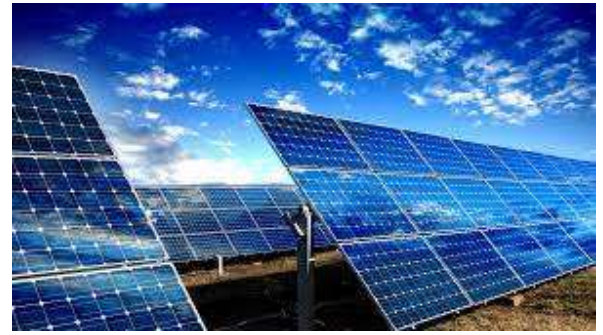
Fig 5. Installation of solar panels(source:google)
